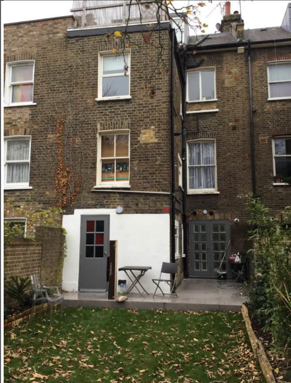
Rear Elevation of 245 Shirland Road
