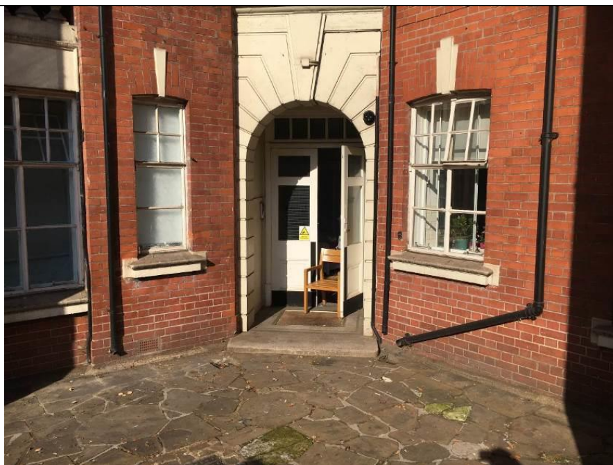
Existing Entrance Doors
